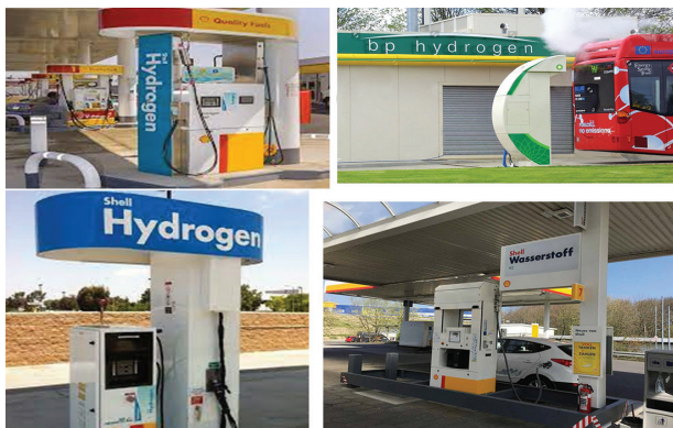
Figure 21. Hydrogen Filling Stations
