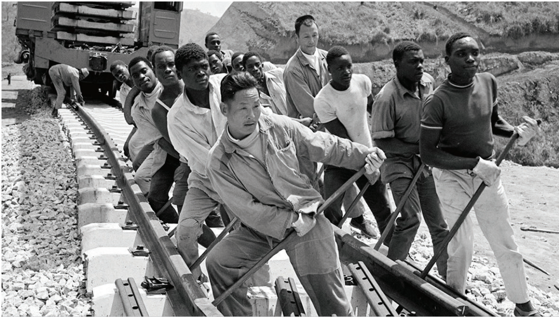
In 1976, Chinese and Tanzanian workers lay track on the Tanzania-Zambia Railway. The 1860.5 km railway is a milestone in China-Africa friendship (Photo: FOCAC, 2016).
