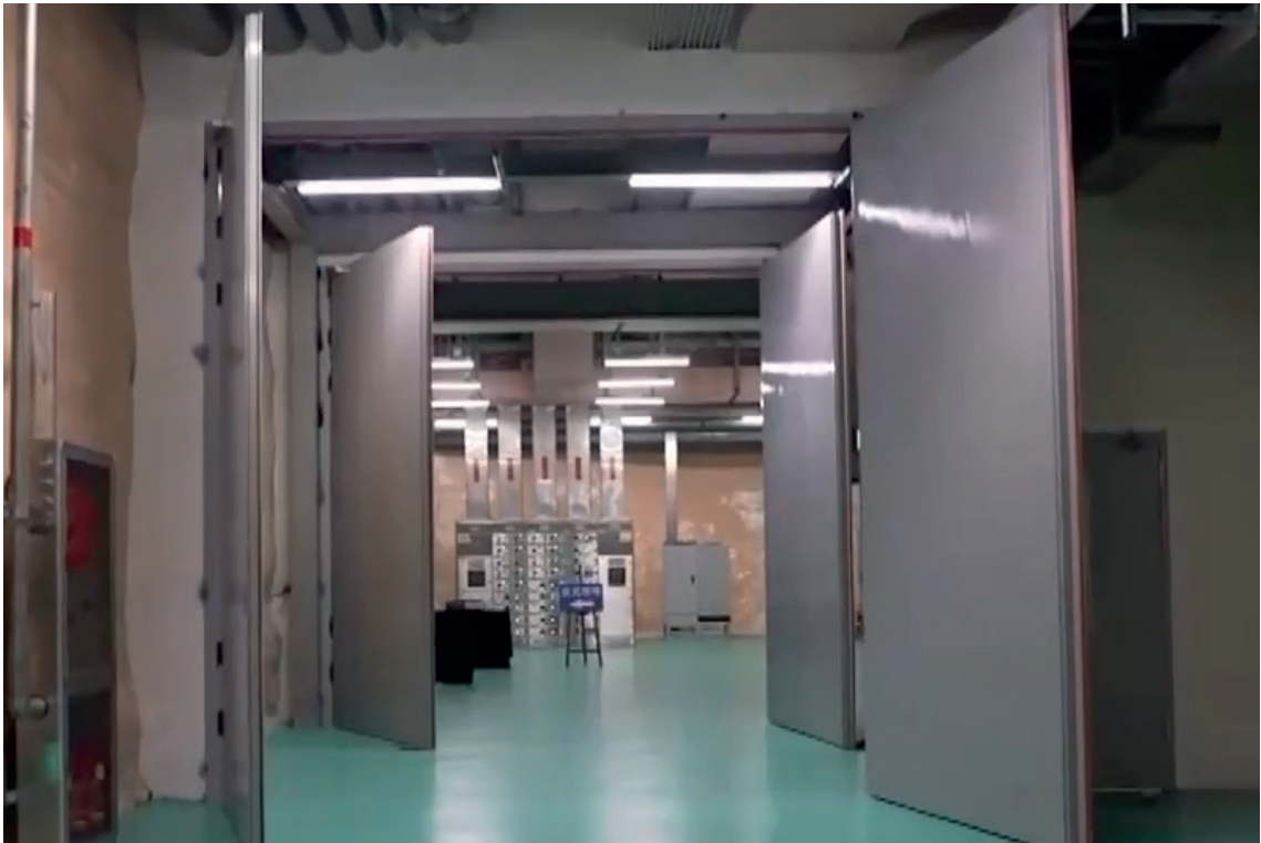
The Deep Underground and Ultra-Low Radiation Background Facility for Frontier Physics Experiments (DURF) is located beneath Jinping Mountain in Sichuan's Liangshan Yi Autonomous Prefecture (Photo: CGTN, 2023).
