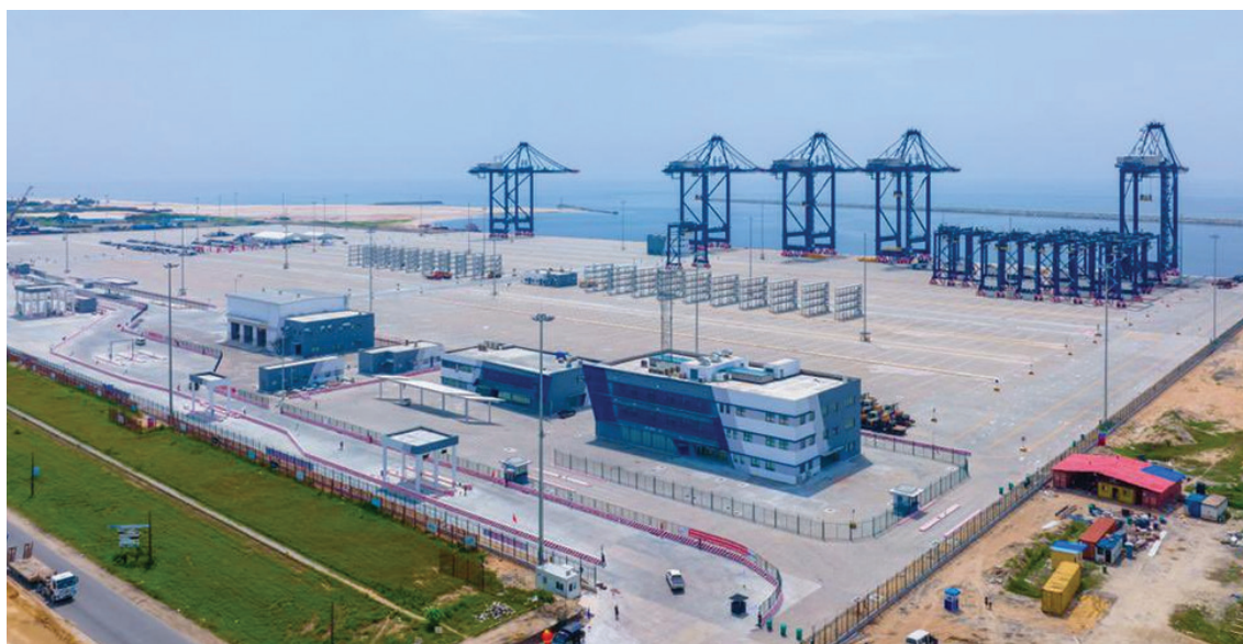
The deepest sea port in West Africa, built by China Harbour Engineering Company Ltd (CHEC) in Lagos, Nigeria (Photo: CGTN, 2023).
