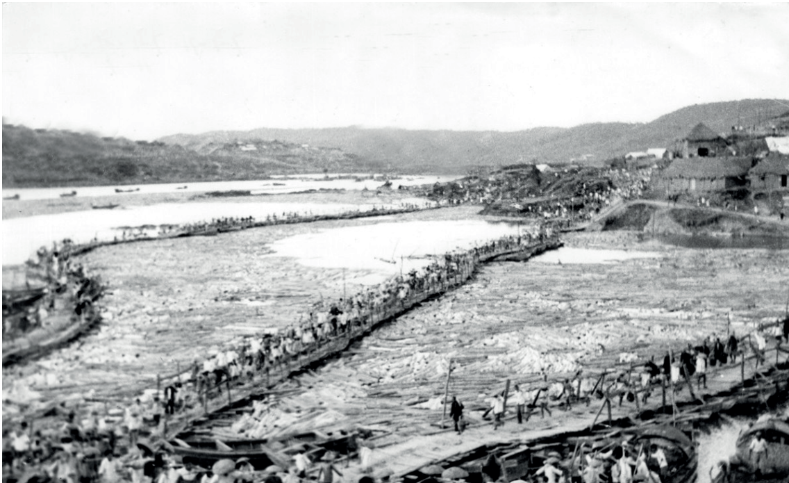
Mass labor mobilization during the Great Leap Forward: building a pontoon bridge to transport earth, Jingmen, Hubei, 1958 (Photo provided by Chen Feng/China Photographers Association, 2021).
