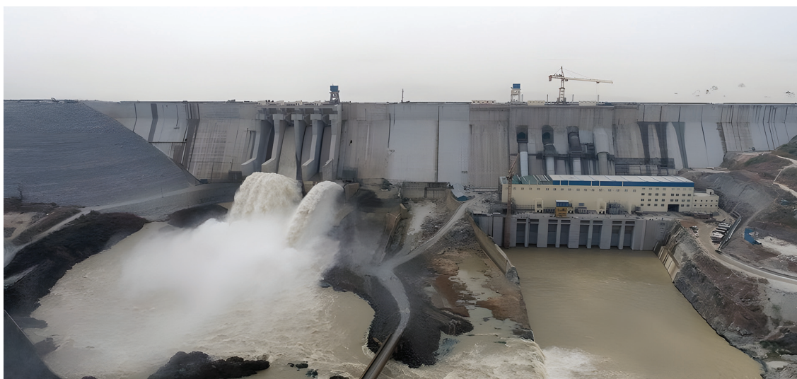
The Zungeru Hydroelectric Power Plant was built by Chinese companies. This plant produces the electricity needs of about 10 percent of Nigeria (Photo: Xinhua, 2023).
