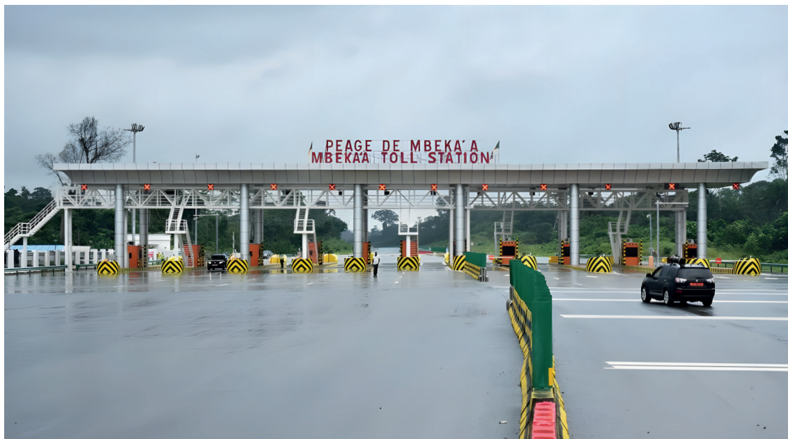
July 2022, Kribi Lolabe Highway, the fruit of close cooperation between China and Cameroon, built by China Harbour Engineering Company Ltd (CHEC) in southwest Cameroon (Photo: Xinhua, 2022).
