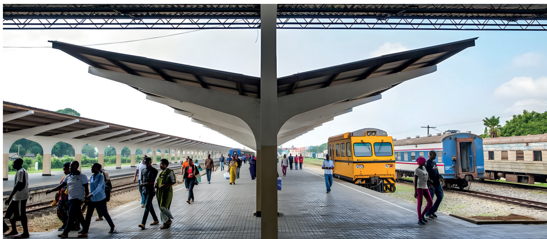
The Dar Es Salaam station of the Tanzania-Zambia Railway in Tanzania on February 14, 2019 (Photo: Xinhua, 2022).
