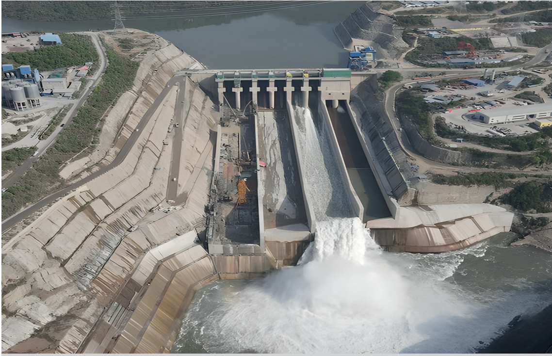
Aerial photo of the Karot Hydropower Project, the first hydropower investment project under the CPEC in Punjab province, eastern Pakistan, April 9, 2022 (Photograph: Xinhua, 2022).
